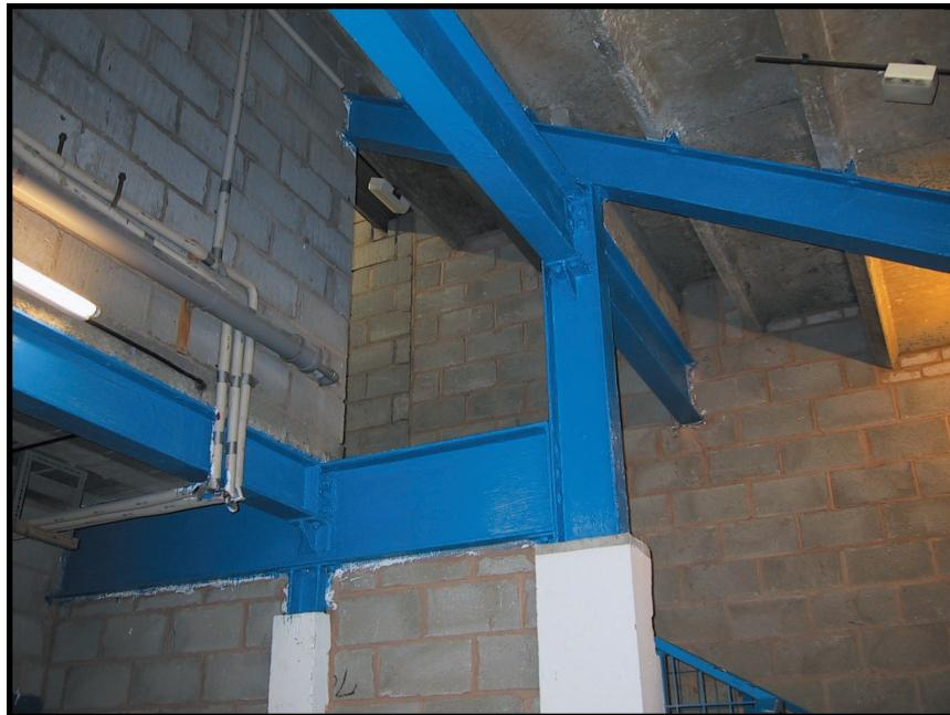
The blast cleaned steel columns and beams were primed with Corro-Tech WB. Our single component, water-based intumescent coating Pyro-Tech SP was then applied to the required micron thickness.
